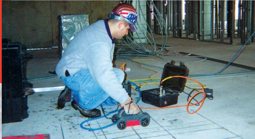
While scanning the area where a penetration is needed, the operator marks the locations of the post tensioned cables
